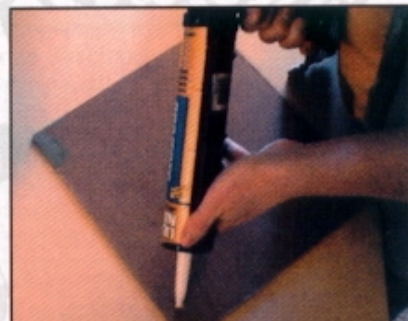
Here we see young Billy "The Animal" Hallam applying some Liquid Nails glue onto the hardboard tile.
