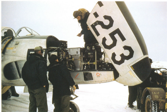
LEFT The working conditions at all bases in South Korea were generally poor for the duration of the war, and harsh winter weather did not help matters. Indeed, the moving parts within the RF-80's battery of cameras were particularly affected by cold and wet weather. Forced to work in the open in near blizzard conditions, these crewmen are seen trying to get film loaded and ready for a mission over the main supply routes in late 1952. The Chinese were using the inclement weather to mask the movement of larger quantities of supplies to the frontline. Once the pictures revealed what the communists were up to, the fighter-bombers were unleashed on the enemy truck columns (Gene Newnam)
