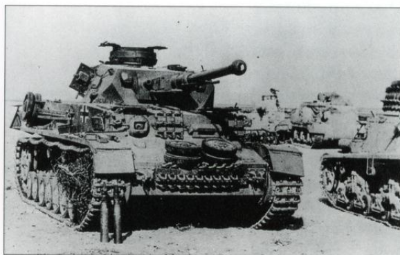
PzKpfw IVF2 captured at Second Alamein; note the size of the two 75mm rounds of ammunition. The tank immediately to the right is an Italian M13/40.
