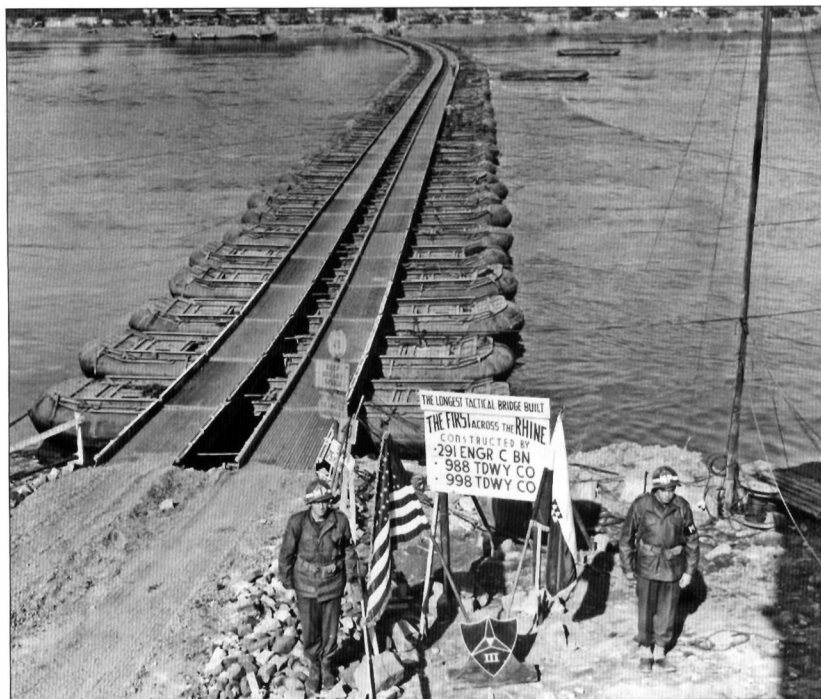
The first of the tactical bridges across the Rhine near the Ludendorff Bridge was a treadway bridge constructed by the 291st Engineer Combat Battalion completed early on the morning of May 11. (NARA)
