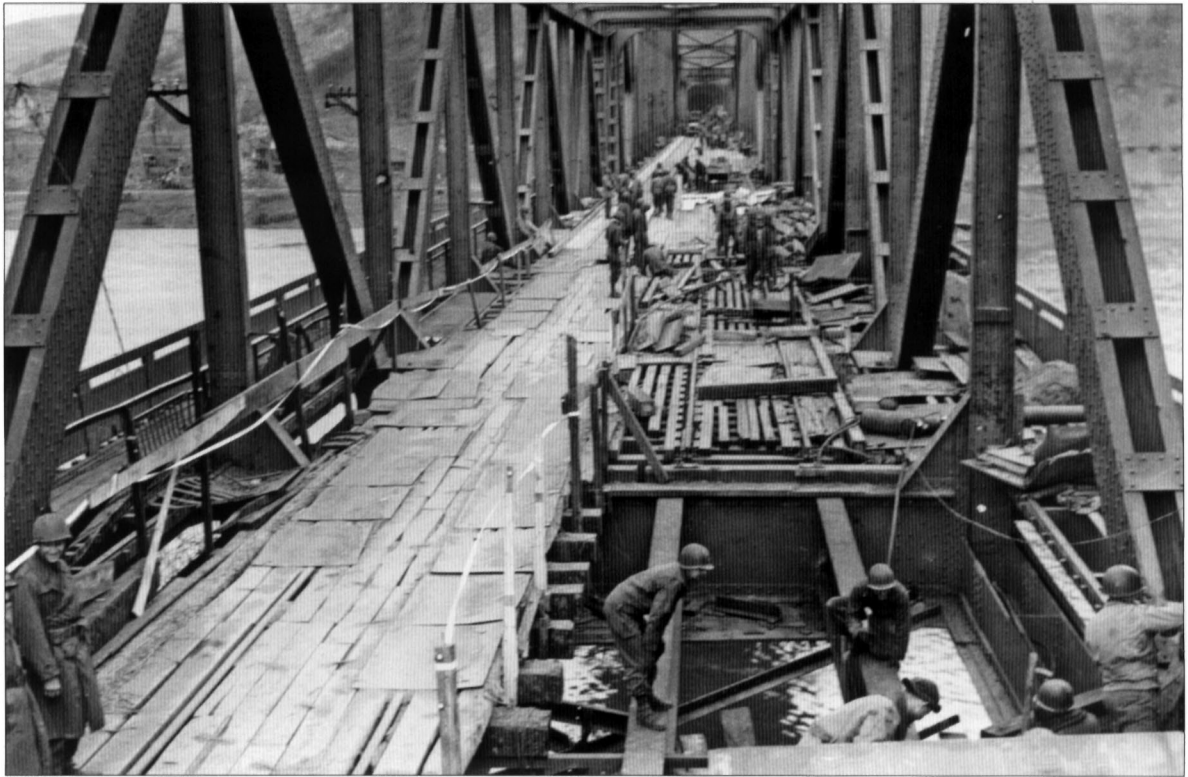
US Army engineers attempt to repair the damage caused to the bridge by the detonation of one of the charges under the eastern pier. This area was further damaged on the night of March 7-8 when a US tank destroyer slipped into the gap while crossing the bridge. (NARA)
