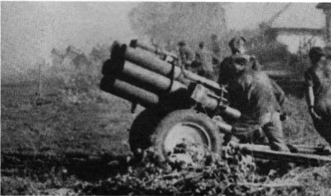
LEFT AND ABOVE: The loading and firing sequence of a 15cm Nebelwerfer – smoke thrower – multi-barrelled rocket launcher. It was developed at the rocket research establishment at Kummersdorf in the 1930s when Germany was banned from building heavy artillery by the Treaty of Versailles. The rocket had a 2.83kg (5.70lb) HE warhead and a maximum range of 7,060m (7,725 yards).
