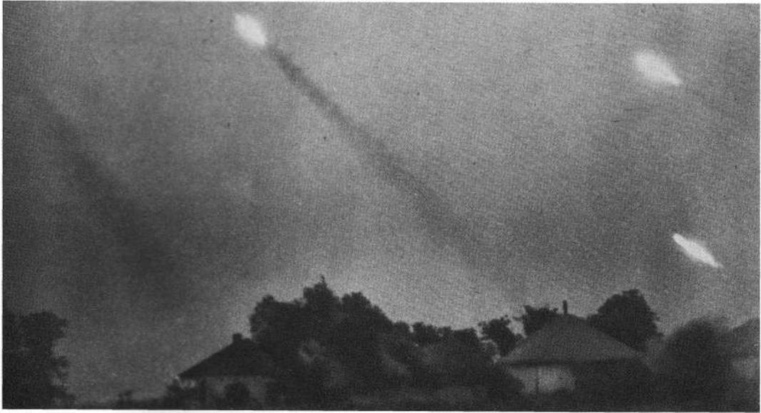
LEFT AND ABOVE: The loading and firing sequence of a 15cm Nebelwerfer – smoke thrower – multi-barrelled rocket launcher. It was developed at the rocket research establishment at Kummersdorf in the 1930s when Germany was banned from building heavy artillery by the Treaty of Versailles. The rocket had a 2.83kg (5.70lb) HE warhead and a maximum range of 7,060m (7,725 yards).
