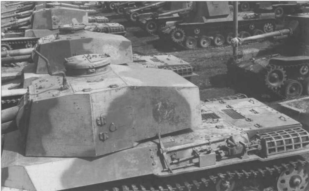
A view of a huge tank park at Hakata, Fukuoka prefecture on Kyushu shortly after the end of the war. In the foreground are some Type 3 Chi-nu medium tanks. Some of the vehicles in the background are the new Type 3 Gun Tank No-ni III, an improved version of the Ho-ni tank destroyer on the Type 97 medium tank chassis, but with a fully armored gun compartment.
