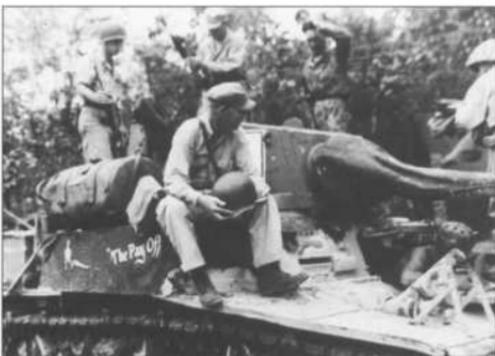
"The Pay-Off", a Marine M3A1 light tank, poses for the camera after landing on Bouganville in the Solomons on 14 November 1943. The two large drums on the rear carry additional fuel. These would usually be dropped before going into combat due to the fire hazard they posed.
