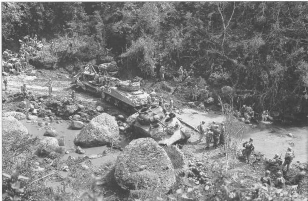
A construction bulldozer from the 117th Engineer Battalion is used to extricate a composite hull M4 of the 775th Tank Battalion that struck a landmine on a small bridge near Baguio, Luzon on 22 April 1945.
