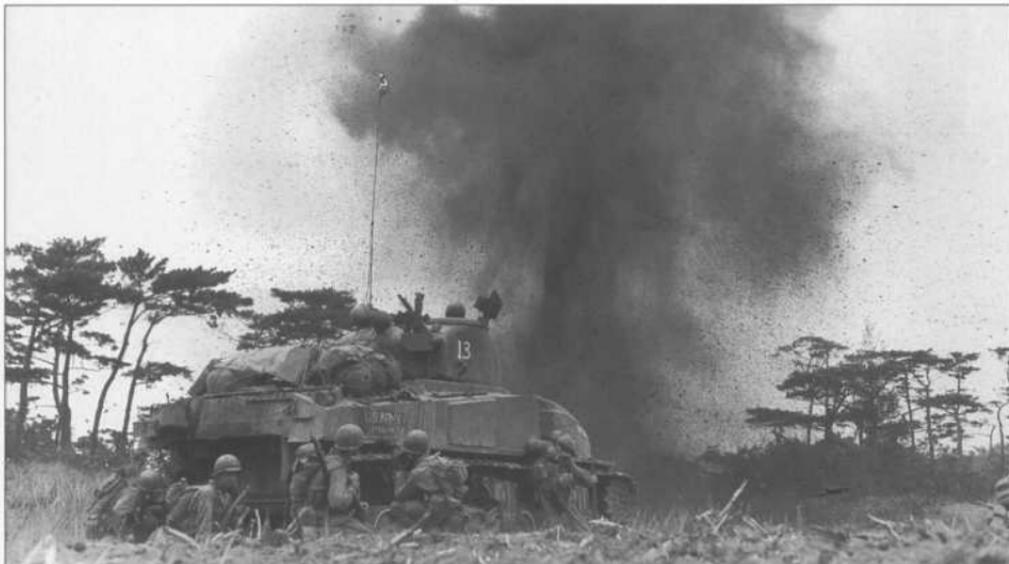
A composite hull M4 medium tank, possibly a flamethrower from the 713th Tank Battalion, comes under fire from Japanese artillery while supporting the 382nd Infantry during fighting on Okinawa on 4 June 1945. Notice the telephone box added on the far left side of the hull rear, a vital new addition to help in tank-infantry coordination.
