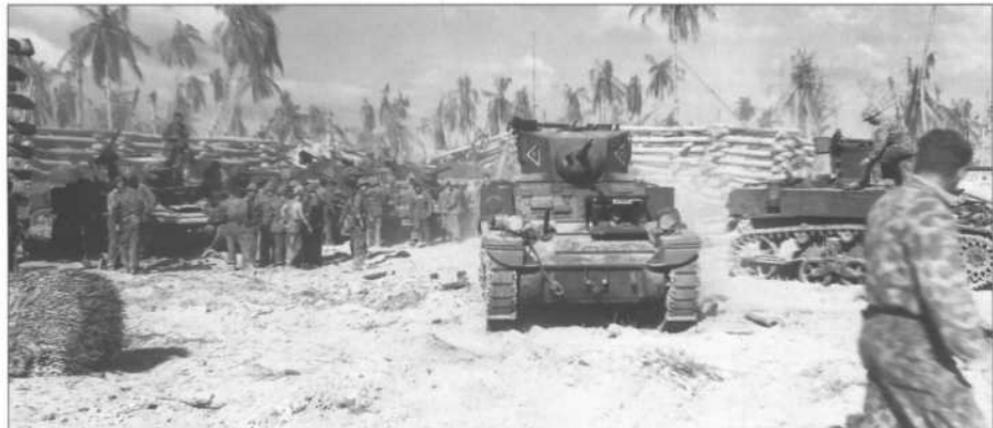
The 2nd Marine Tank Battalion took over a stockade area on Betio and established a repair and refueling area during the final mop up operations on the island. The battalion used a triangle insignia to indicate the companies, pointing up, down and to the side to indicate different companies.
