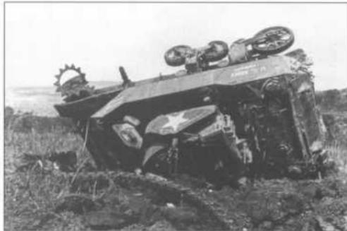
One of the most deadly enemies of tanks on Saipan were mines. The Japanese occasionally used aerial bombs along likely tank routes. This mine has managed to blow off the front right bogie, snap the drive sprocket, and knock the tank over.
