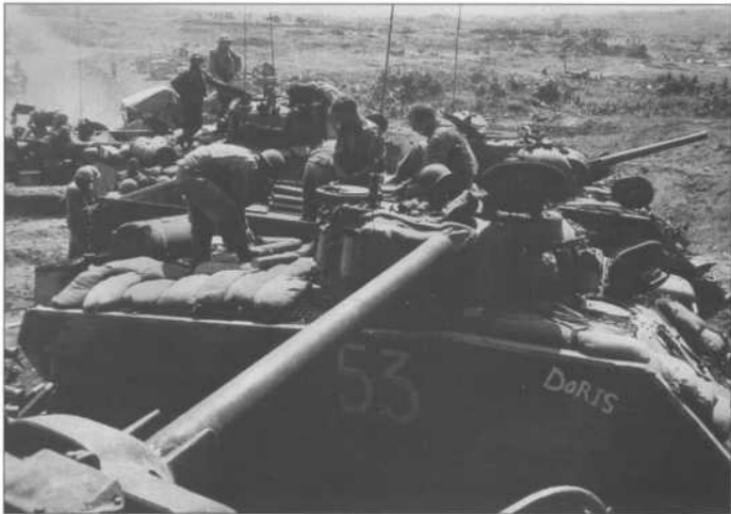
"Doris", a M4A2 (W) of the 4th Tank Battalion, is resupplied with ammunition from trucks. This gives a good view of the metal grating fixed over the engine deck area to act as stand-off protection from Japanese satchel charges. The extra spacing was intended to give the explosives room to vent, minimizing the damage transmitted to the tank.
