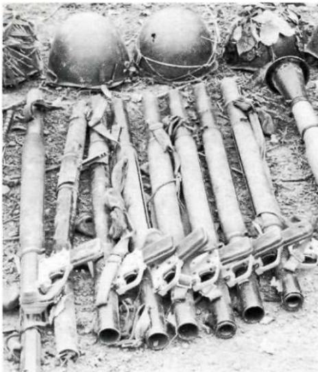
*Russian-manufactured rocket-propelled grenades (RPGs) were the descendants of the very successful Second World War German hand-held anti-tank weapons. Nominally effective up to 500 yards, in combat the NVA and VC employed RPGs at*
