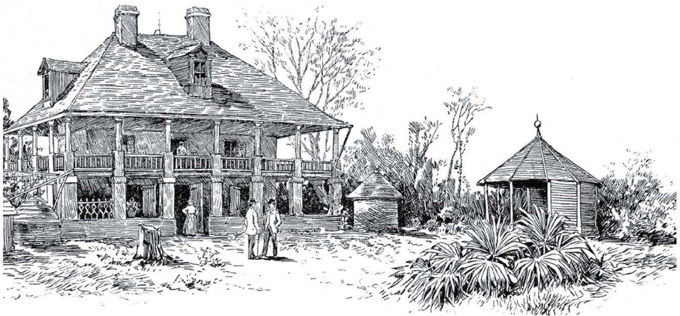
Louisiana Plantation House
