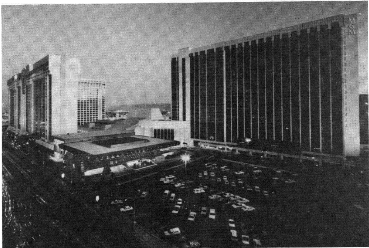
Exterior of the MGM Grand Hotel.
