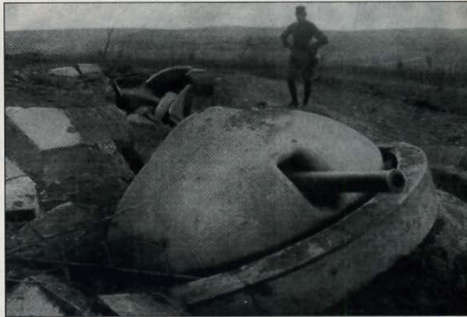
Results of the second bombardment of Przemysl — broken towers on Fort No. 10.
